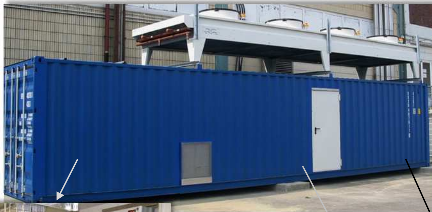
R404A multi temperature refrigeration plant integrated in a 40 ft
