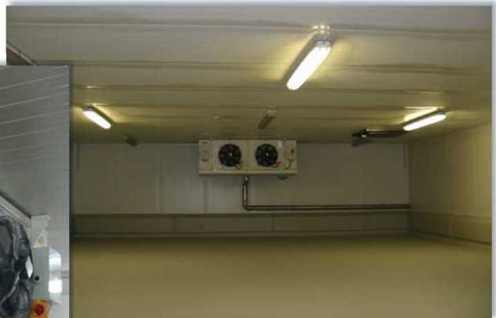
R404A evaporator in the cooling rooms
