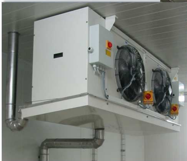
R404A evaporator in the cooling rooms
