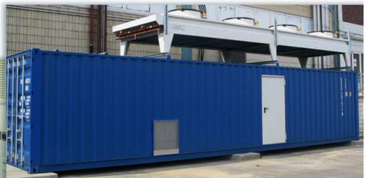
Ten production and storage rooms are maintained at different temperatures using an air-cooled R404A dual purpose refrigeration system.
