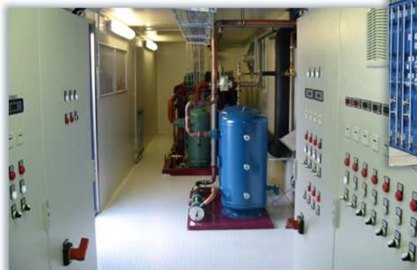
Ten production and storage rooms are maintained at different temperatures using an air-cooled R404A dual purpose refrigeration system.
