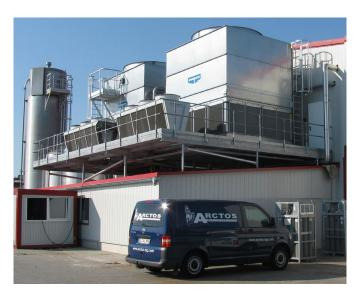
Evaporator and cooler of the NHM / COM cascade refrigeration system on a steel platform near the machine room. Below are the cooling water facilities, heat recovery components, and water treatment system.
