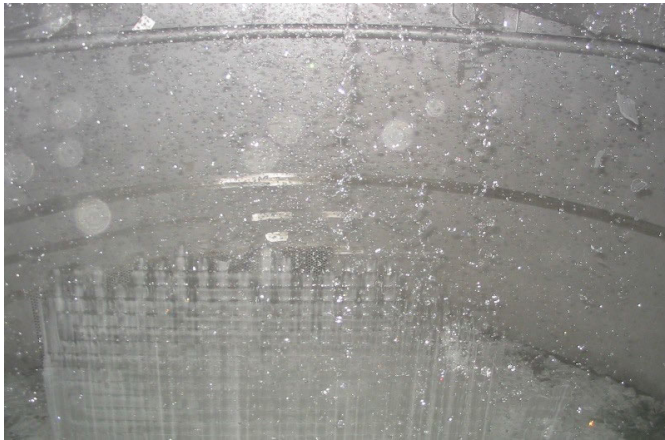
Inside the Ice Water Silo in Operation (Production of Crushed Ice)
